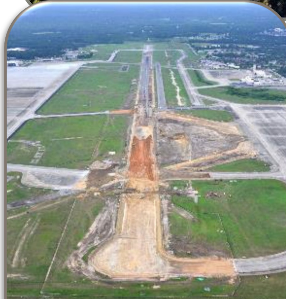
Pope Army Airfield Runway Replacement
